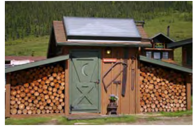
Solar Powered Outhouse
